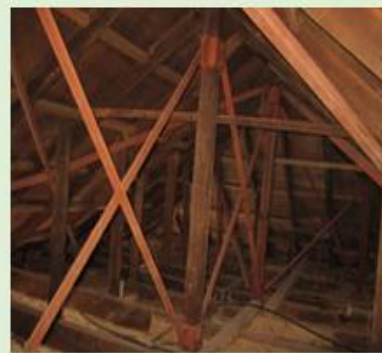
Steel bracing to roof
