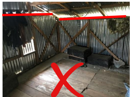
Discontinuous top plate at different level
